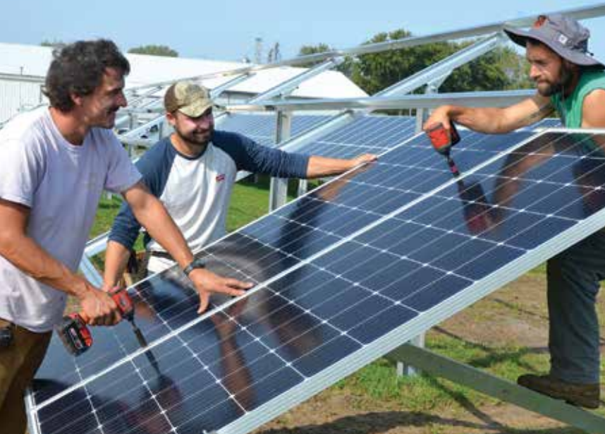
Alumnus Chase Grabau '17, Logan Wood '18 and Cory Thielen '16 (l-r) install one of the 684 solar arrays now located adjacent to the University's Peacock Arts and Athletic Center. The solar project is expected to generate approximately 70% of the electricity demand of the PAAC and Harms-Eischeid football stadium.
